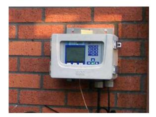
Figure 3-14 Signature Flow Meter mounted on wall
