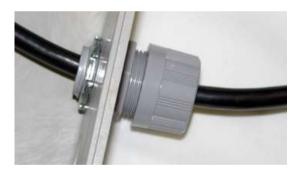
Figure 2-10Position and secure the cable
